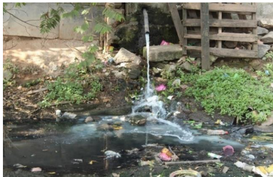
11. Unsafe drainage system in urban area (Photo credit: Dhanushaka Disanayaka)
