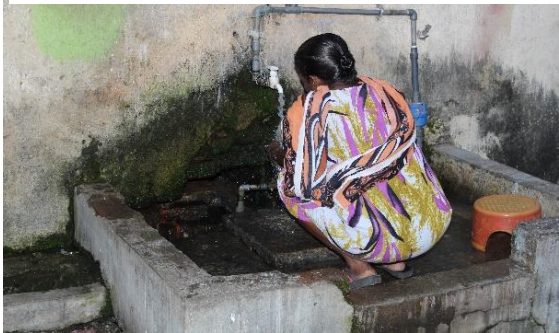
13. Public pipeline in urban slum areas (Photo credit: Dhanushaka Disanayaka)
