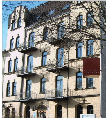
Front of the INCHER-building, Mönchebergstrasse 17, Kassel
