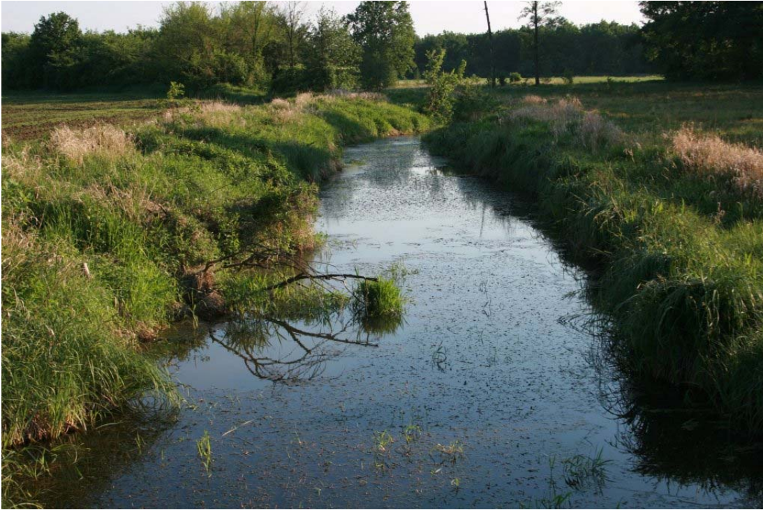
Figure 33. A well-maintained ditch of the Land Reclamation System in the Odra region.
