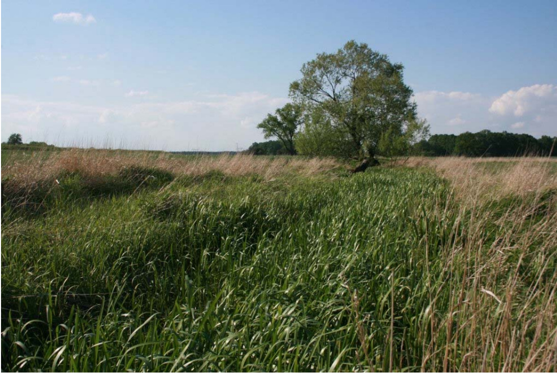
Figure 32. A neglected overgrown ditch of the Land Reclamation System in the Odra region.
