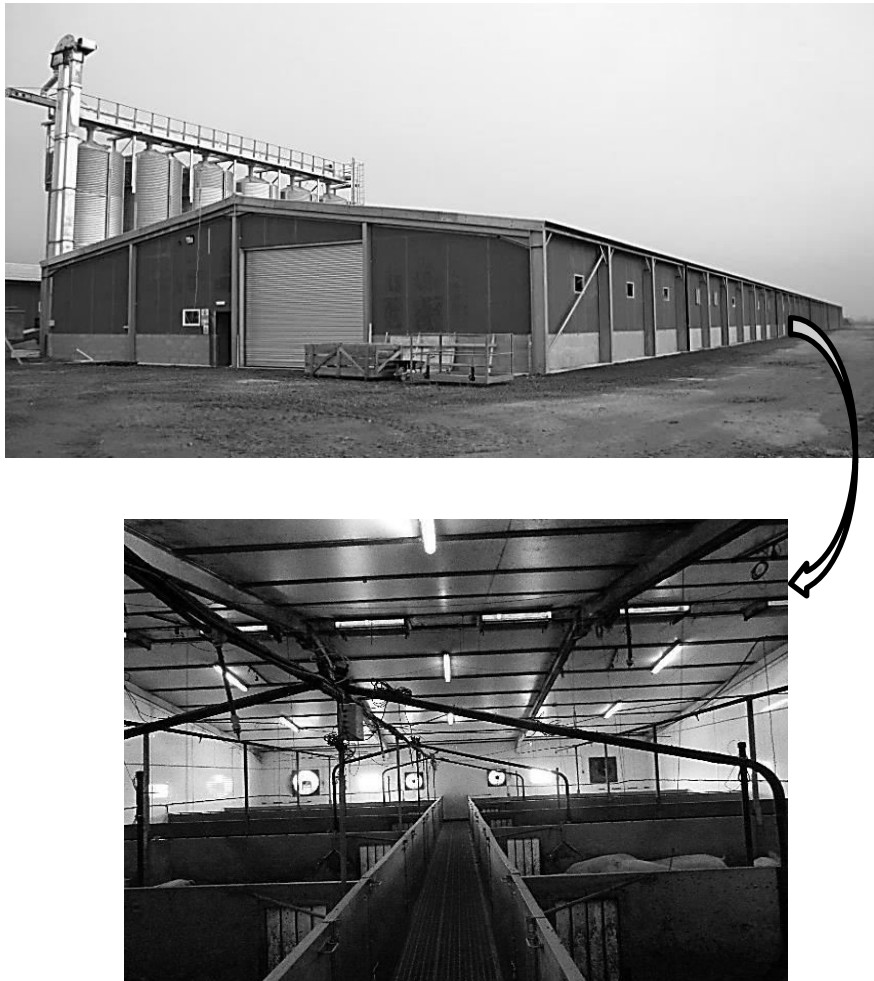
Figure 4.1- External view of the commercial barn (top) and internal view of a research room (bottom).
