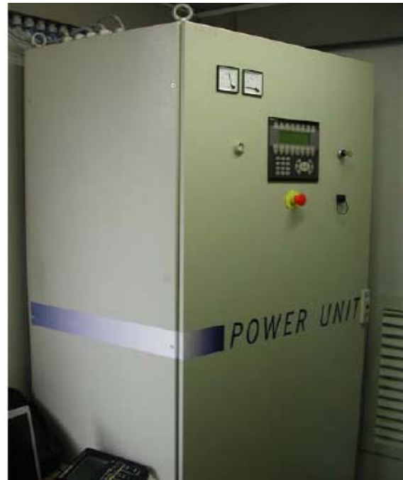
The alkaline Electrolyser 3.6kW (Hydrogen Systems) and the PLC Box from Hydrogen Systems, www.hydrogensystems.be
