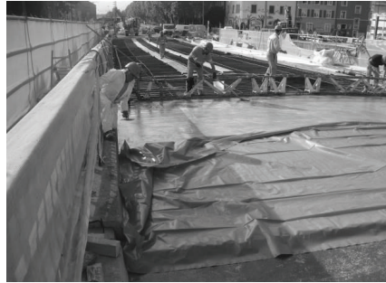
Figure 4: UHPFRC overlay paving
