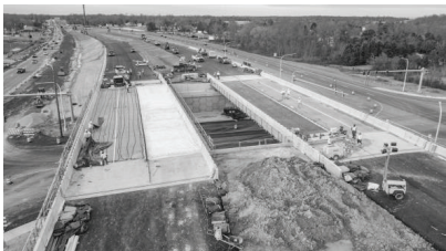
Figure 3: SR1 Bridges during Construction
