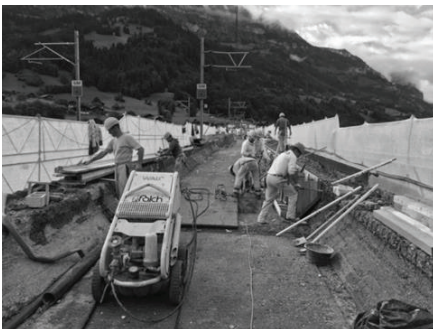
Figure 1: Preparation work for UHPFRC
