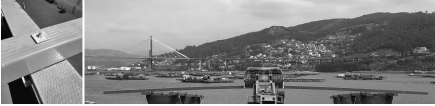
Figure 2: Detail of a connection (left) and placing of a beam (right)
