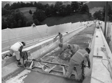
Figure 2: UHPFRC paving
