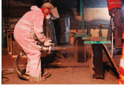
Figure 1: UHPFRC spraying
