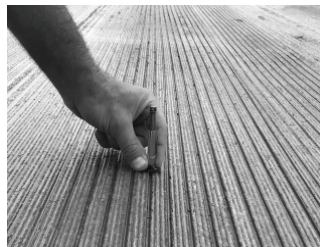
Figure 2: Diamond grooved UHPC overlay surface
