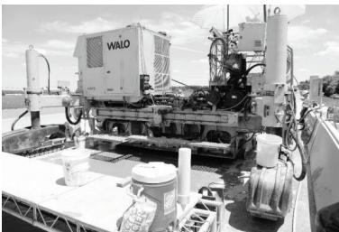
Figure 1: Fully mechanized paving machine
