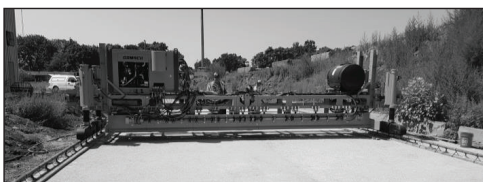
Figure 5: Highly Specialized Thin Lift UHPC Paver
