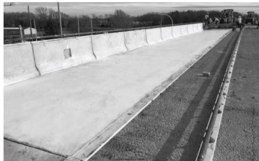
Figure 4: UHPC Overlay after Stage #1
