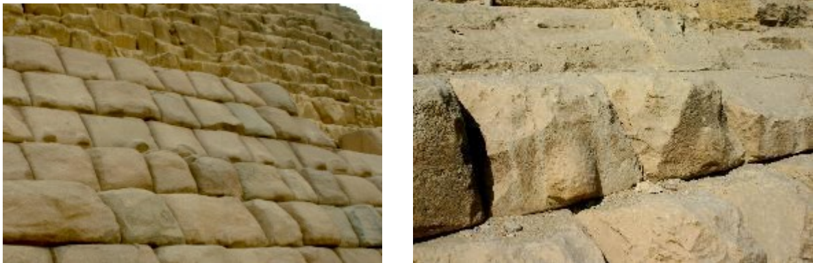
Fig. 3. Bosses on the facade blocks of the Mykerinos Pyramid (left) and one of Cheops' side pyramids (right) bear witness to the fact that, they were lifted into position. (photos by U.E. Dorka)
