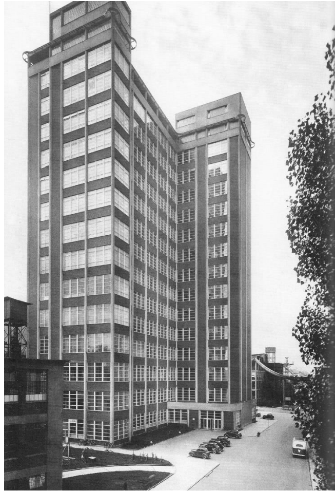
Figure 21: The Bata administration building in 1938. 104
