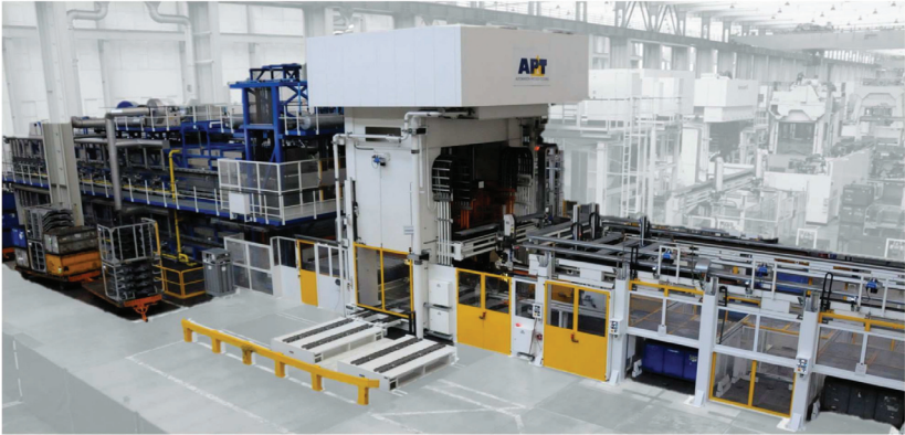
Figure 1.2.: A hot stamping line with two stacked heating furnaces (left) and the press in the picture's center. The picture was taken at the Volkswagen plant in Baunatal.
