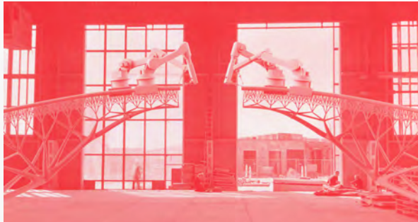
Joris Laarman & Heijmans: robots building a 3D-printed bridge over an Amsterdam canal
