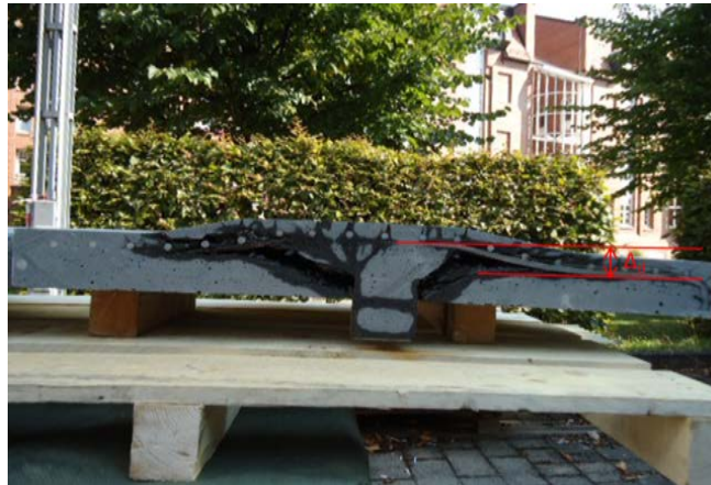
Fig. 4.6: Deformation of reinforcement bars due to dowel action
