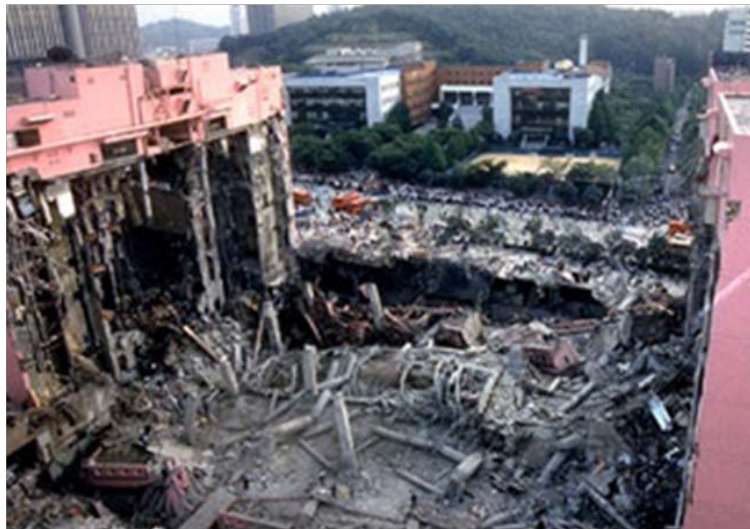
Fig. 1.2: Post-collapse photograph of the Sampoong Department Store
